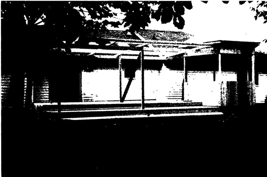
Figure 1. The Gazebo Observatory under construction.
